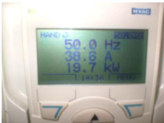
When things go wrong or short cuts are required to overcome issues unrelated to drives there can be a philosophy of 'put it into hand and run at 50Hz'. Whilst this may overcome immediate problems if forgotten the drive is then not performing at its optimum level and can be wasting significant quantities of energy. Therefore just ensuring that the drive is operating under auto or remote control can lead to significant savings .
